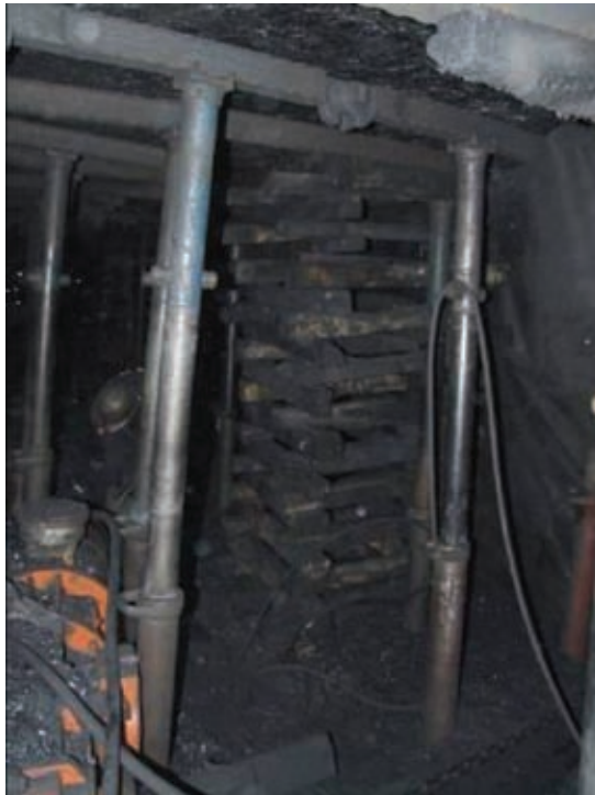
Figure 5-7: Hydraulic Props and Cog Support at the Operating Working Face
