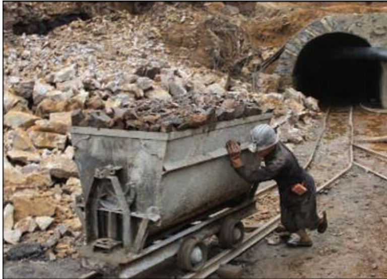
Figure 5-2: Construction of new Incline at Xinghe in Progress
